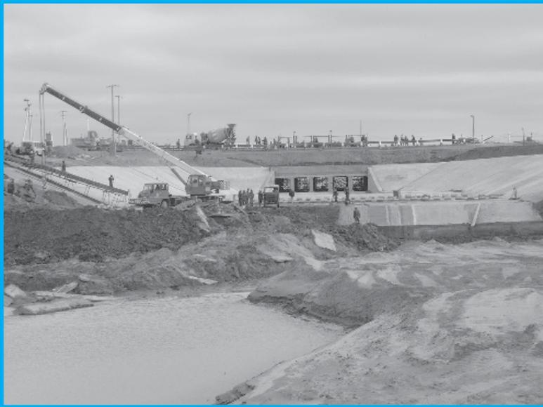
**Last works on Aitek dam reconstruction, in the Karaozek area, operated by the Chinese Geo-engineering Corporation. The maximal flow in the Syrdarya will be raised from 300 m<sup>3</sup>/s to 700 m<sup>3</sup>/s.**
