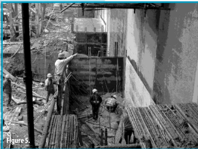
**Figure 5. Construction of concrete blocks at the heel of the dam below low level cracks.**
