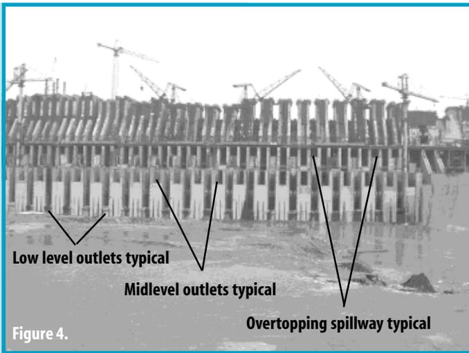
**Figure 4. A photo of the downstream face, during the flooding of the downstream area, showing the three levels of outlets.**
